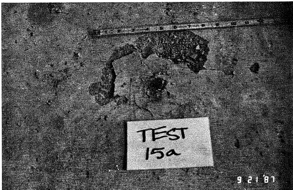
Fig. 6.2 Mode 1 Behavior (Shank Fracture, No Slip) for Adhesive and Grouted Anchors
